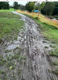
There is another section further west where the bank on the north side of the bridge has been washed away near Harvton Street. The bikeway has been completely cut due to damage caused by the flood.
