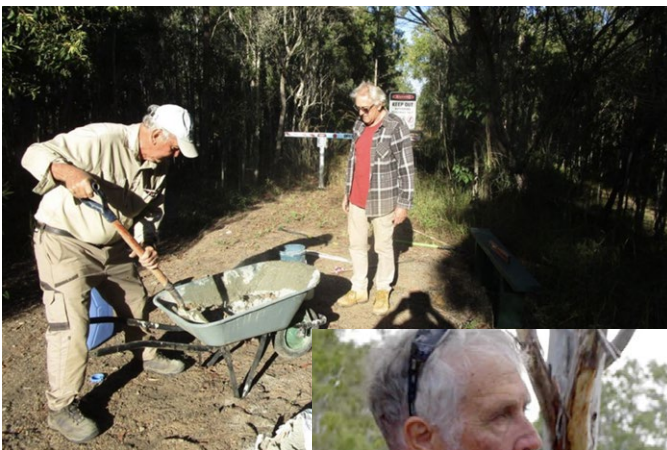
Volunteers Ken and Wayne, installing seats at Bridges 3, 4, and 5.
